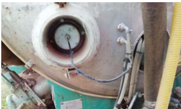
Conductivity meter installed in the transport tank
