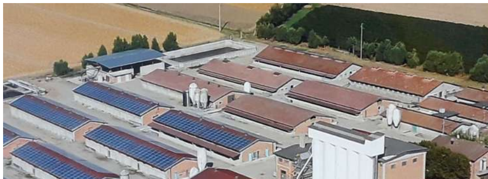
Sant'Anna pig farm, partners of the Gas Loop operational and experimental site
