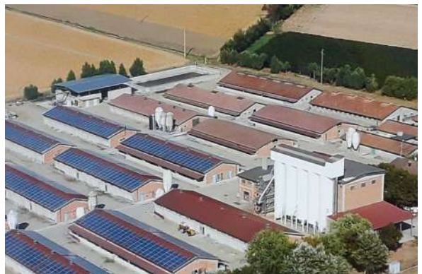
Sant'Anna pig farm, partners of the Gas Loop operational and experimental site
